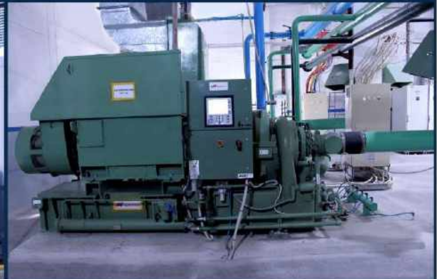
INGERSOLL RAND TA3000 / TA6000 Air Compressor (670 KW)
