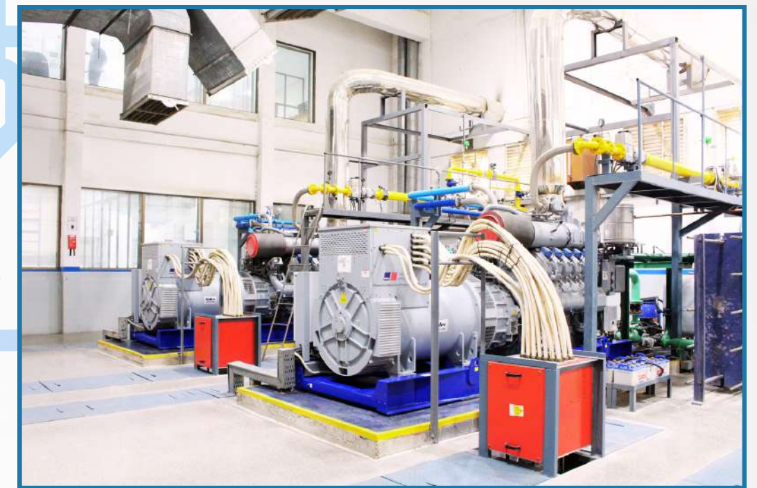
MTU 12V 40lciaL64 Gas Generator (1521 KW)
