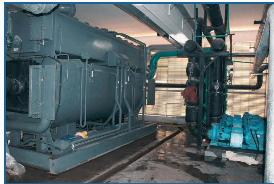
Absorption Chiller 360 USRT
